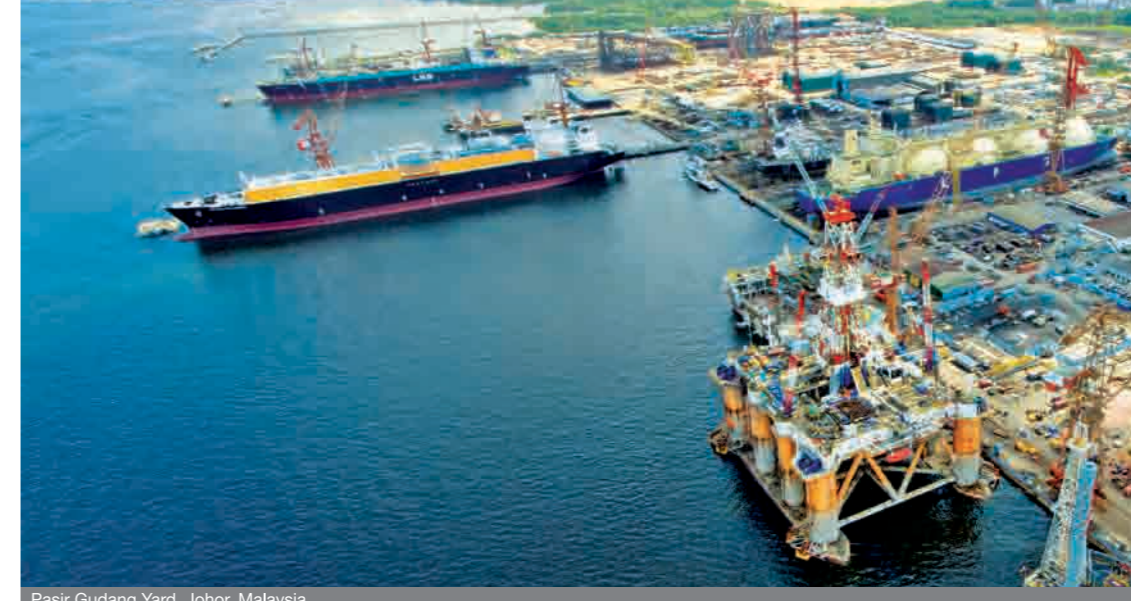
Pasir Gudang Yard, Johor, Malaysia
