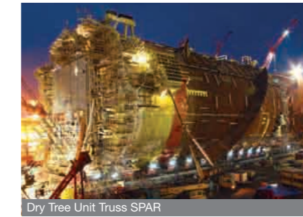
Dry Tree Unit Truss SPAR
