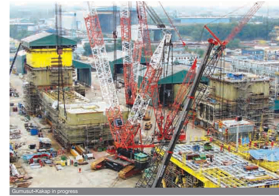
Gumusut-Kakap in progress
